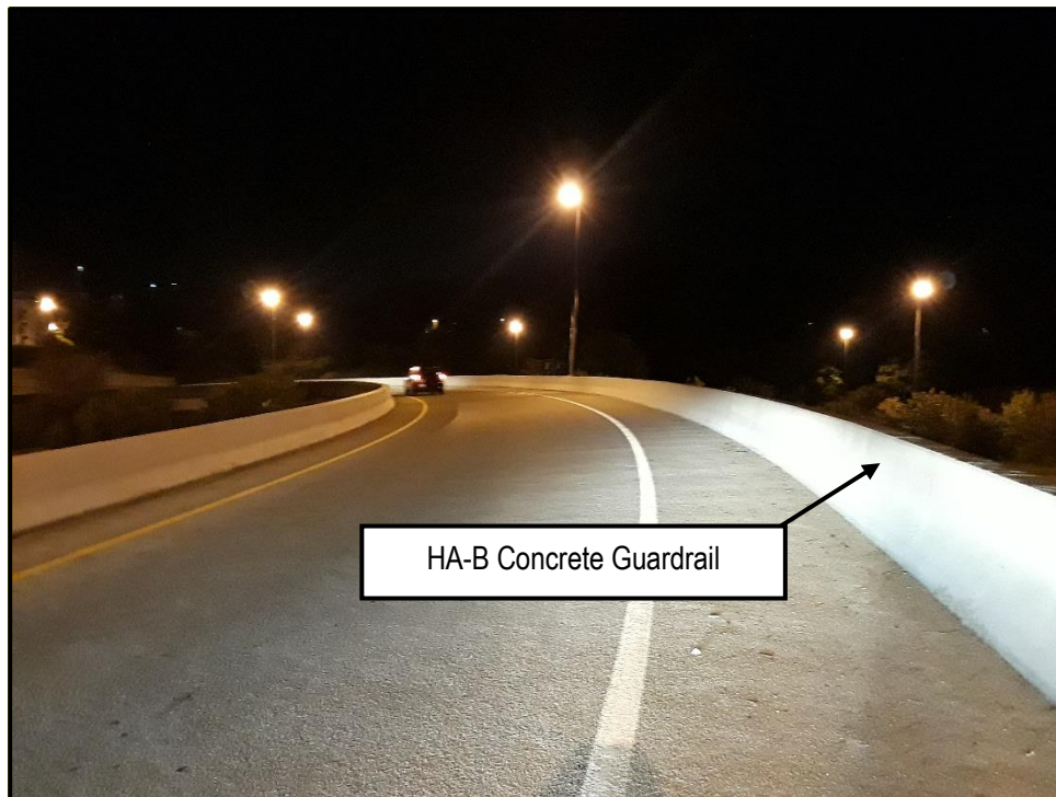
Photo 2: View of HA-B on the SR-1 Ramp over I-440
