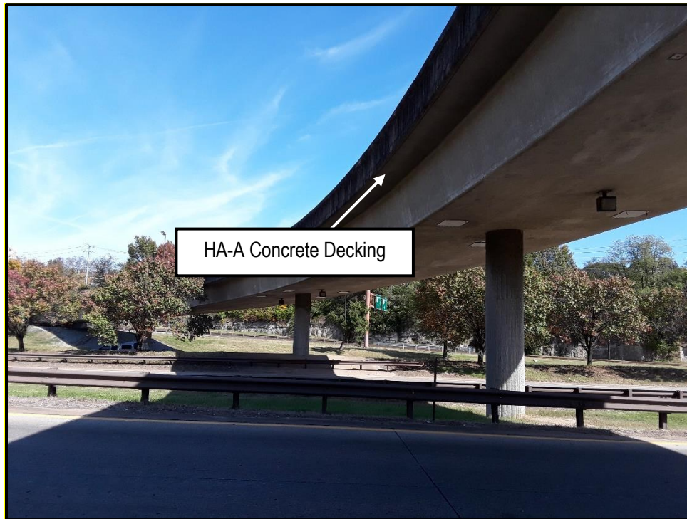
Photo 1: View of HA-A on the SR-1 Ramp over I-440
