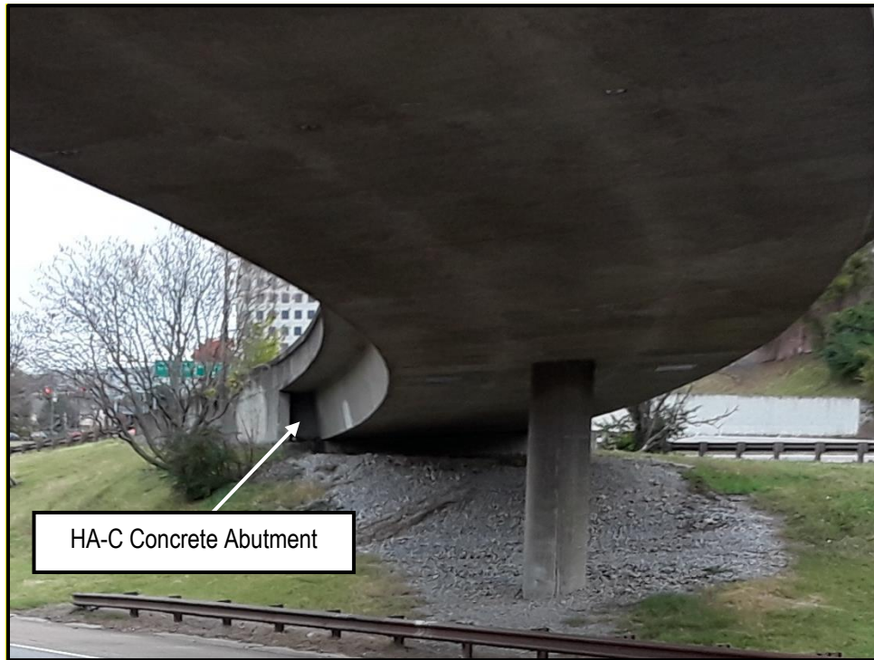
Photo 3: View of HA-C on the SR-1 Ramp over I-440
